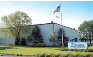
UST Sandusky Plant
