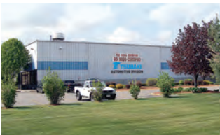
UST Chicopee Plant
